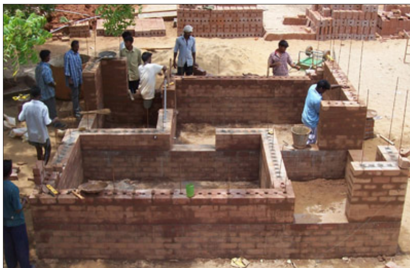
Low Cost Shelter being built.
